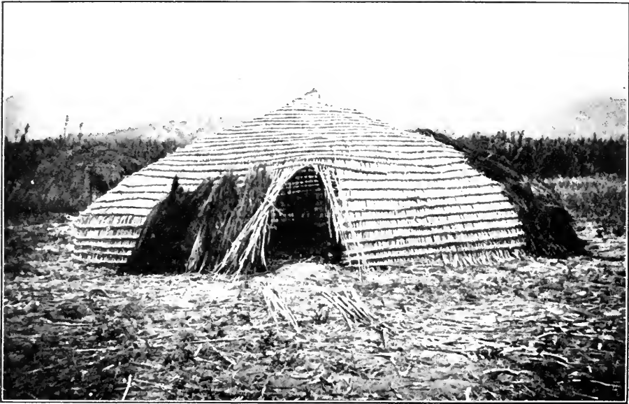
A HUT FRAME AT BAWIRA
